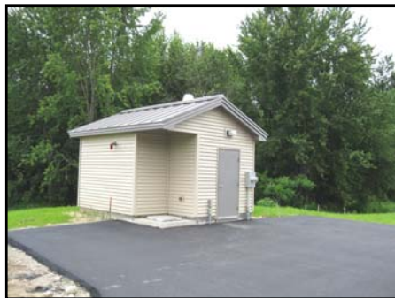
New West Farmington Pump Station
